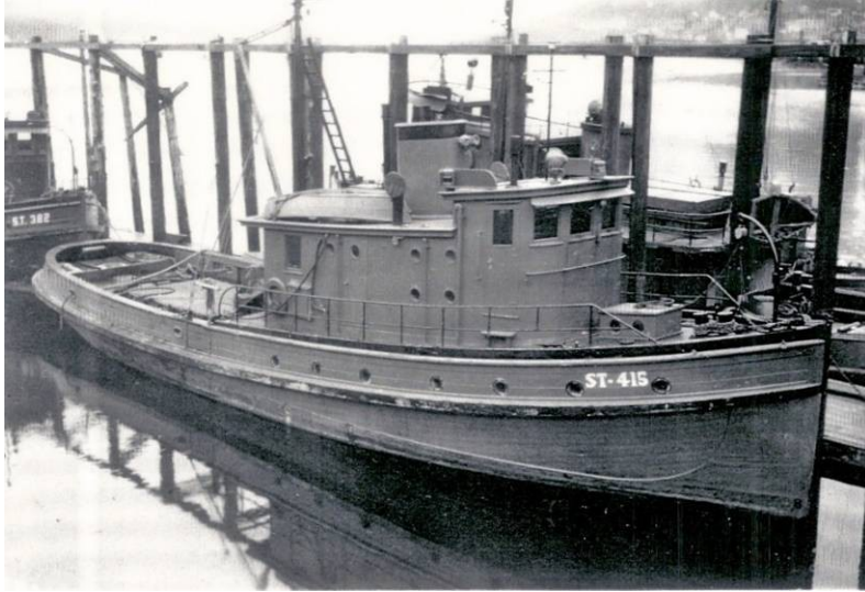
ST 415 with a replaced superstructure, a common mod on early ST's due to weight issues
